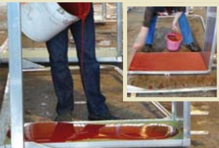
Boards with 13 mm(!) thick plastic filling and granulate spread on!
